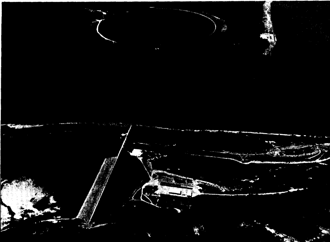
Figure 2-17. Seneca off-stream pumped-storage project, which uses the Allegheny Reservoir behind Kinzua Dam as its lower reservoir (Courtesy Pennsylvania Electric Company and Cleveland Electric Illuminating Company)
