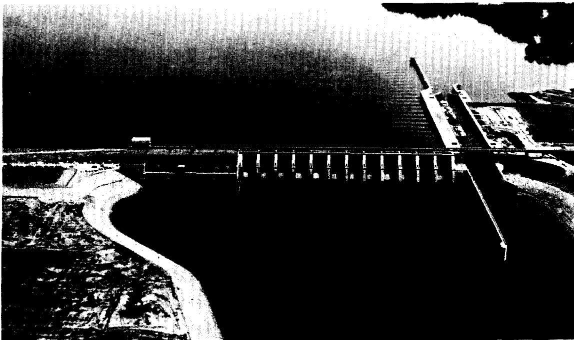
Figure 2-15. Barkley Lock and Dam, a run-of-river project with pondage (Nashville District)
