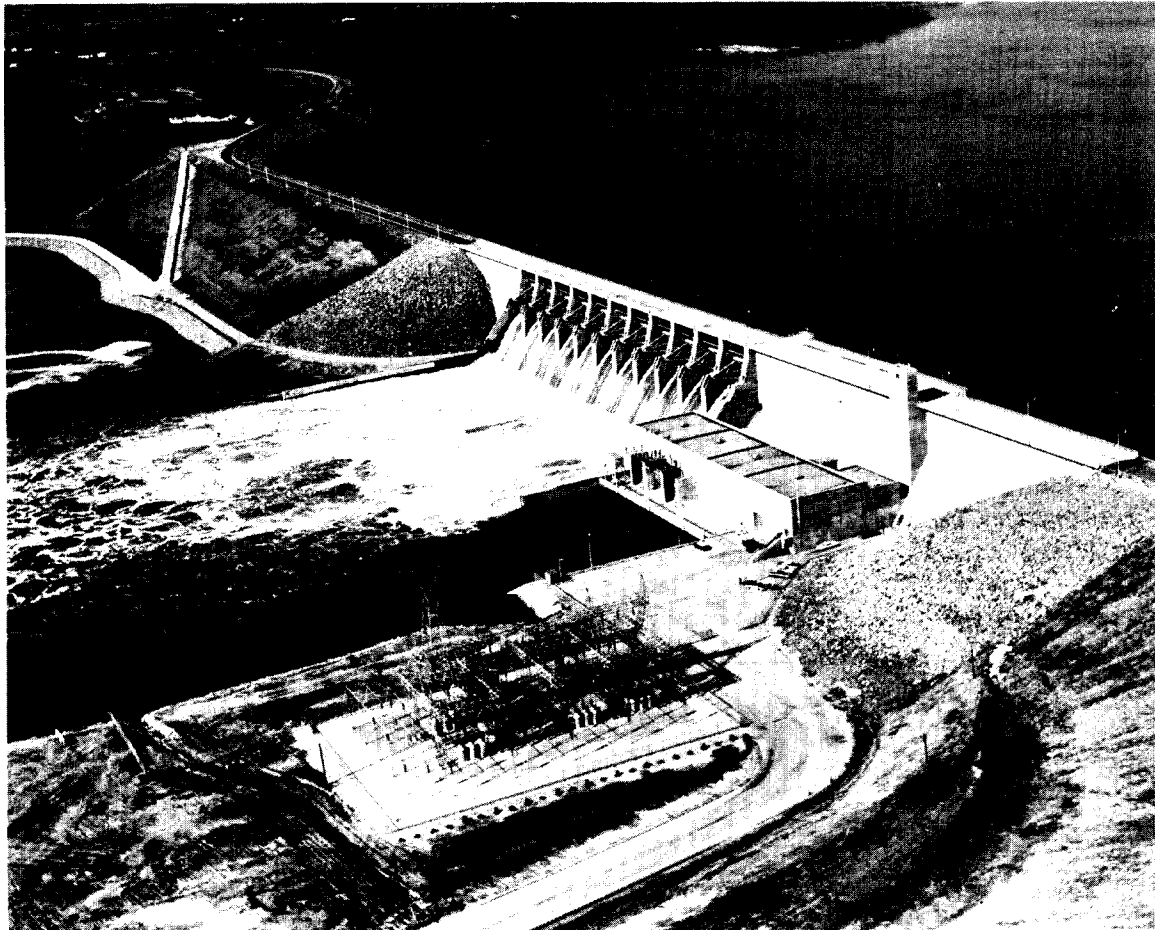
Figure 8-4. Eufaula Dam and Lake (Tulsa District)
