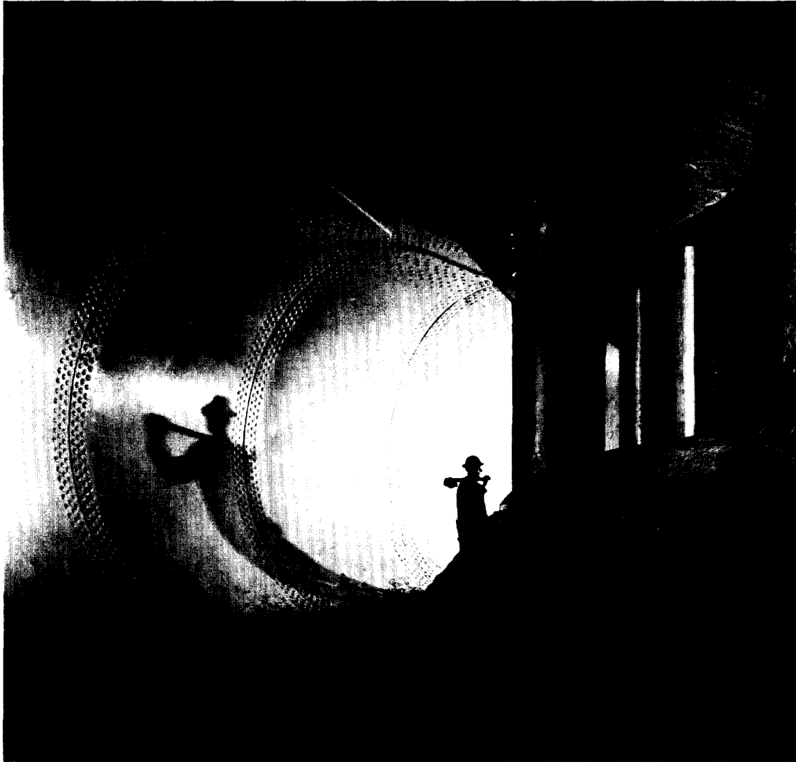
Figure 2-28. Spiral case and wicket gates, Norris Dam. This is an older plant (1936) featuring riveted rather than welded construction, but the photo dramatically illustrates the shape of the water passageway (Courtesy of Tennessee Valley Authority)
