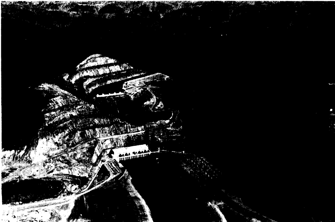
Figure 2-18. Carters pump-back project (Mobile District)
