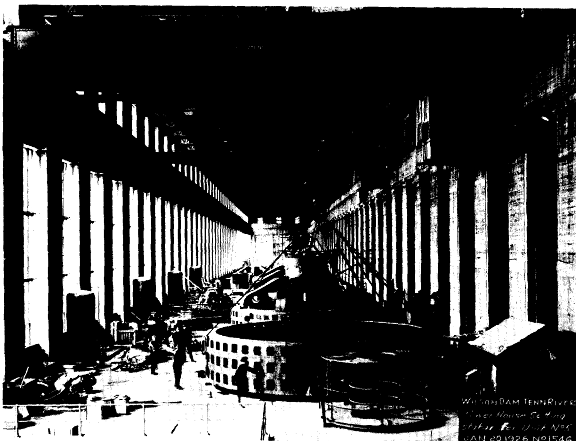
Figure 1-2. Generator installation at Wilson Lock and Dam, the first major hydroelectric project to be designed and constructed by the Corps of Engineers. The project was placed in service in 1925 and was transferred to the Tennessee Valley Authority in 1933 (Nashville District).
